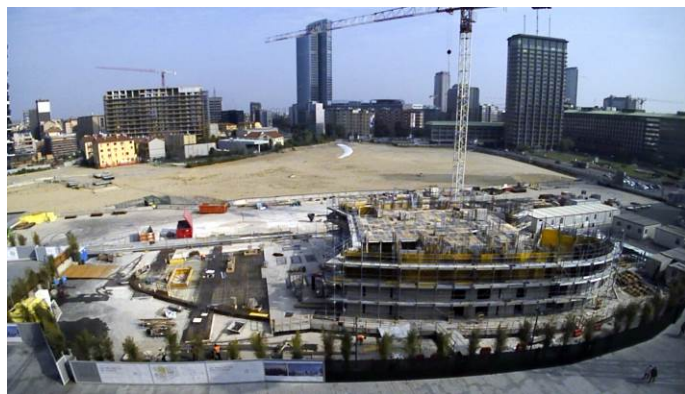
Figure 7. View of concrete core walls and foundation / vista muri di controvento e fondazione in c.a.
