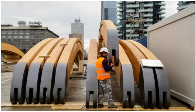
Figure 24: storage area for wood laminated beams on site / area di stoccaggio travi lamellari in cantiere.
